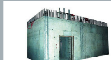
A vault room after filling with concrete mixture and de-panelling
