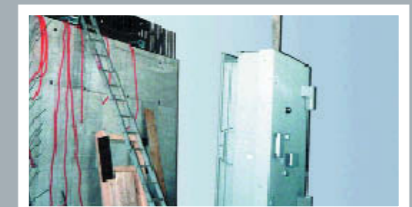
Installation and assembly of vault door
