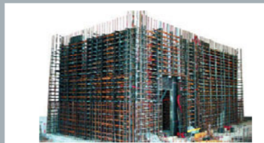
Armoring elements and static armoring elements of a vault room, prepared for panelling and filling with concrete mixture
