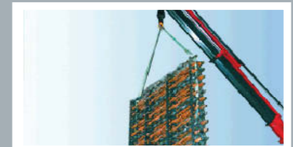
Installation and assembly of wall armoring elements
